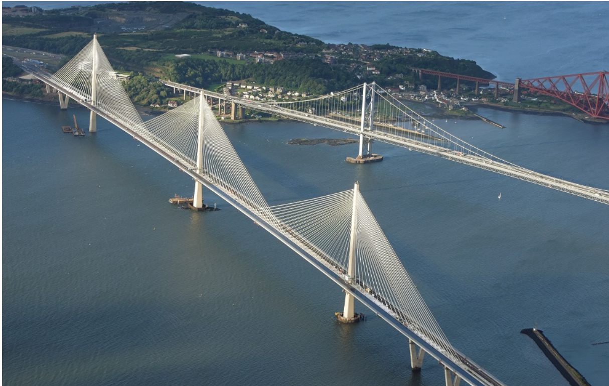
Figure 4.6: Queensferry crossing (left, cable-stayed), the Forth Road bridge (middle, suspension) and parts of the Forth bridge (right, red steel truss). Courtesy of: Scottish Construction Now.
