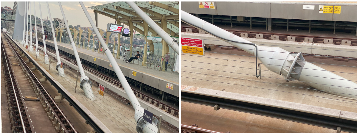
Figure 2.7: Cable anchorage tubes of a railway bridge in Istanbul, Turkey.
