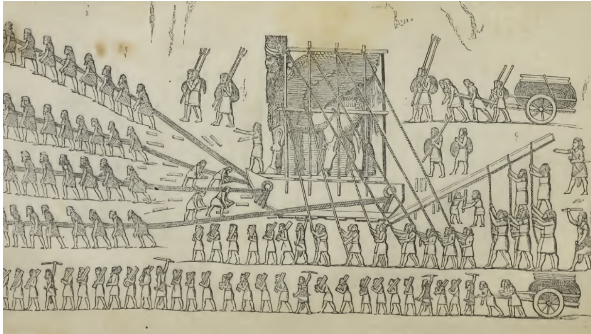
Figure 1.2: Using rope in construction and lifting of heavy object, utilising the lever arm concept in Assyrian civilisation about 1800 B.C. (Courtesy of A. H. Layard's Nineveh and Babylon 1859).
