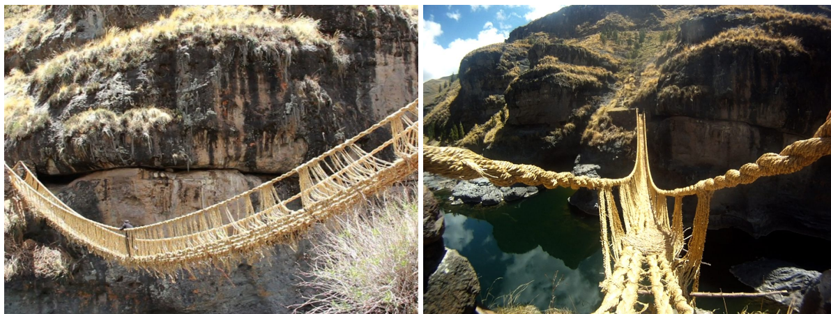
Figure 1.4: Q'eswachaka bridge crossing the Apurimac canyon in Peru and a close-up of its main straw-woven suspension ropes.
