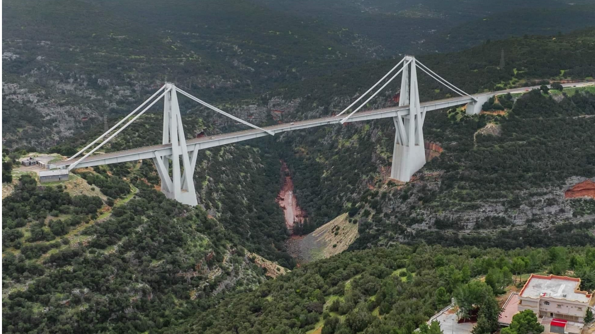
Figure 1.5: Wadi el Kuf bridge near Al Bayda, Libya. Courtesy of: Sanad Al-Ahlafi.
