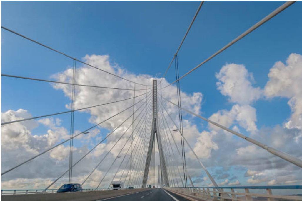
Figure 2.11: Cross ties connected to stay-cables of the Normandy bridge in France. (Courtesy of David Henry - Getty Images).
