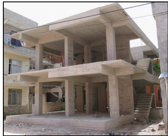
(b) Building STR1 (under construction)
