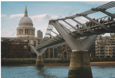
(c) Millenium Bridge, London [5]
