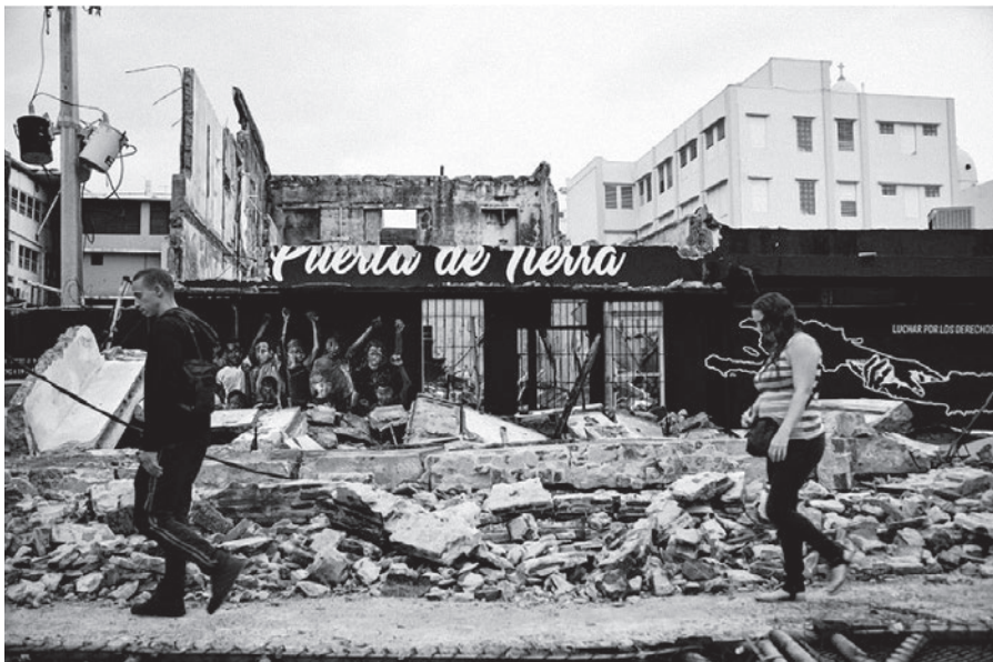
Fig 3: Puerto Rico destruction after Hurricane Maria.
