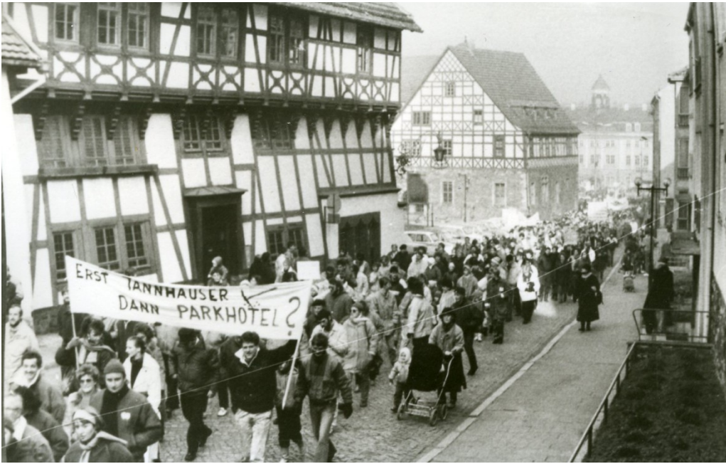
Figure 5-12 Demonstration against Demolition of Tannhäuser (1989), Eisenach Stadtarchiv
