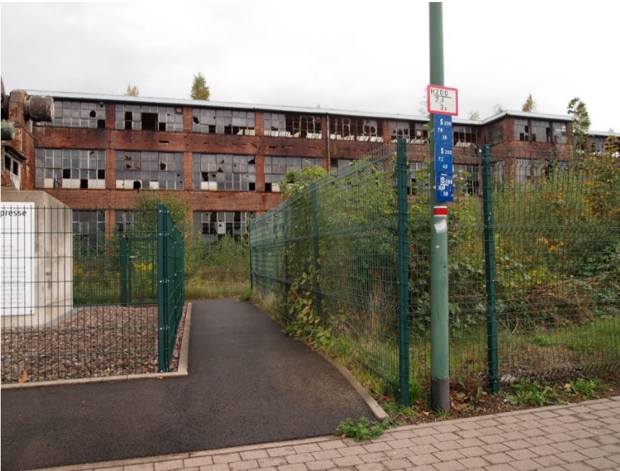
Figure 5-17 Former AWE building (Sung, 2015)
