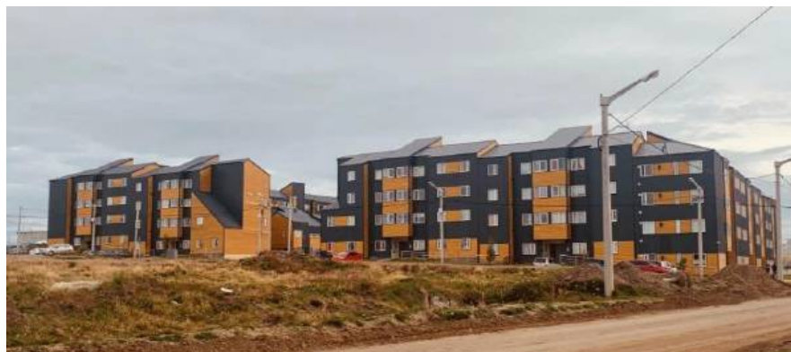
Figure 6.40: PROCREAR dwellings, multifamily complexes. Río Grande. Source: own records
