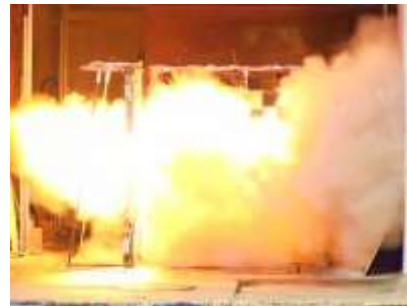
Fig. 9 View of the switchgear during internal arc fault test
