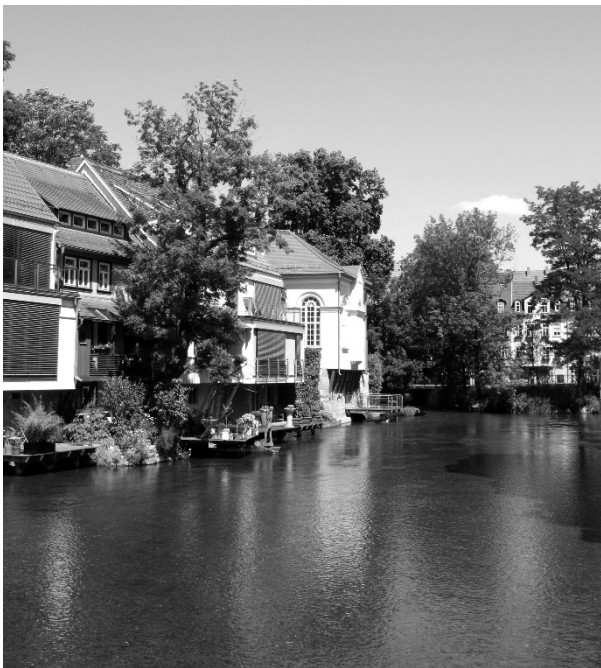
Figure 2. 19th century synagogue with built-in mikva on the Gera. – Reformsynagoge mit Mikwe im Keller an der Gera. Photo by authors.
