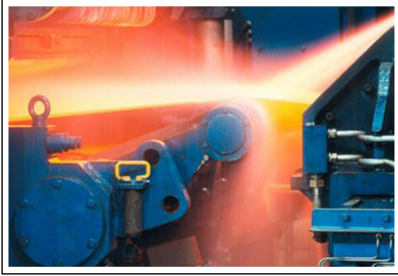
Figure 3. Looper system between rolling stands.
