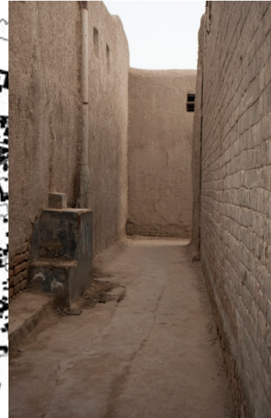
Figure 4.7: Narrow streets of Bhitshah old neighbourhoods, varying between 3' to 8' with minimum openings.
