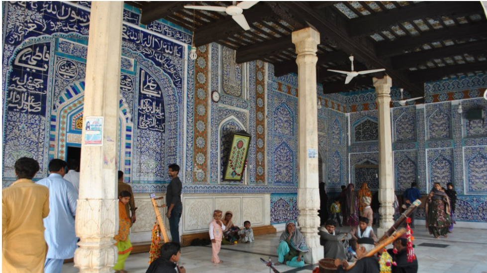
Figure 5.16: Entrance porch of the tomb entrance showing kashi tile work, carved wooden beams and monolithic marble columns
