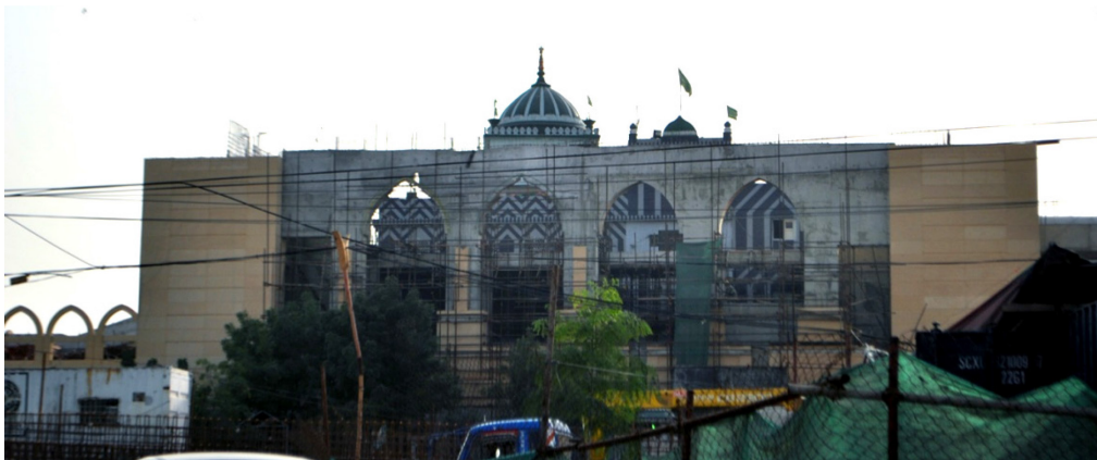
Figure 5.11: Shrine of Abdullah Shah Ghazi under construction
