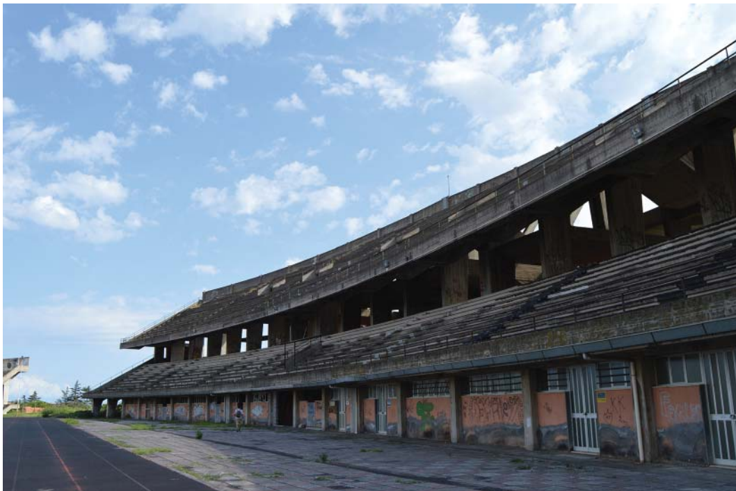
Fig. 1. Athletics Stadium and Polo Field, Giarre Source: Pablo Arboleda, 2015
