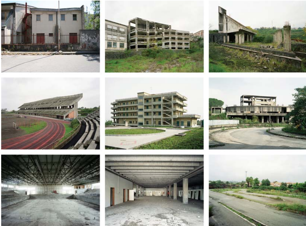
Fig. 2. Unfinished public works in Giarre. From left-right and top-down: New Theatre; Multi-storey Car Park; Children's Park; Athletics Stadium and Polo Field; Care Home; Multi-functional Hall; Olympic Swimming-pool; Flower Market; Radio-controlled toy-car track. Source: Alterazioni Video, 2008
