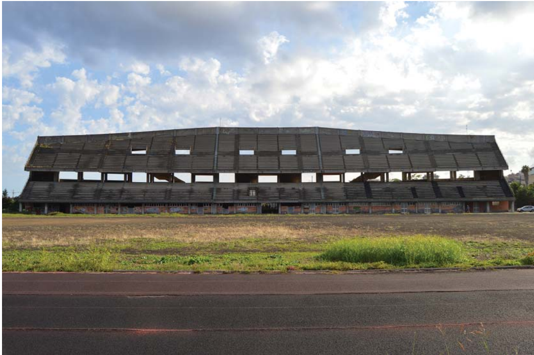
Fig. 2. Athletics Stadium and Polo Field, Giarre Source: Pablo Arboleda, 2015
