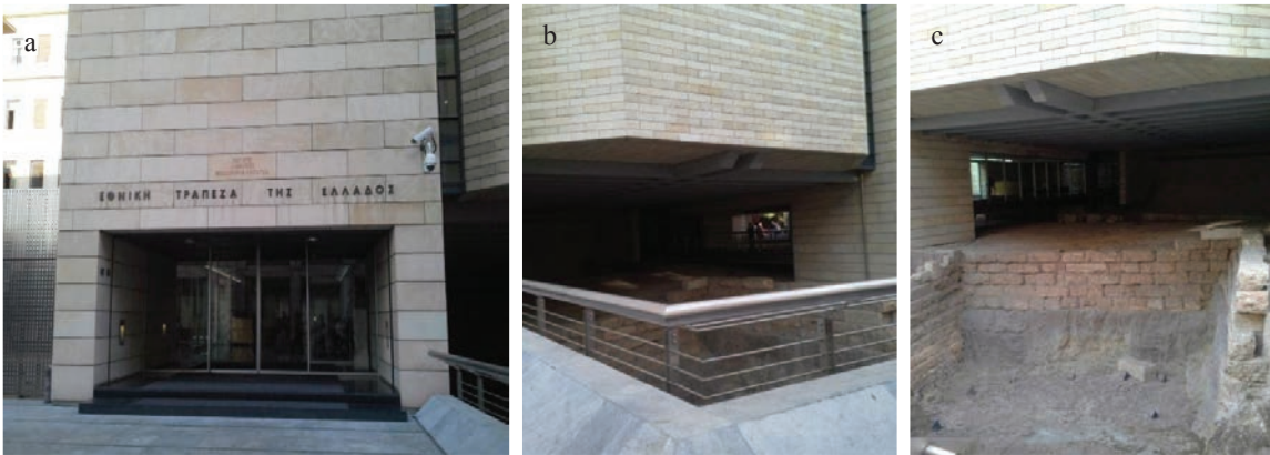
Fig.7.(a) Eonikh Tpaneza building Façade with main entrance, Athens, Greece; (b)(c)The archeological part under the building. June 2015.Source: Researcher
