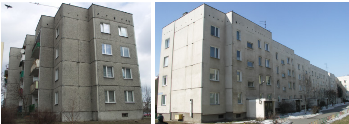
Fig. 1. Examples of large – panel residential buildings with old facade (Warsaw)
