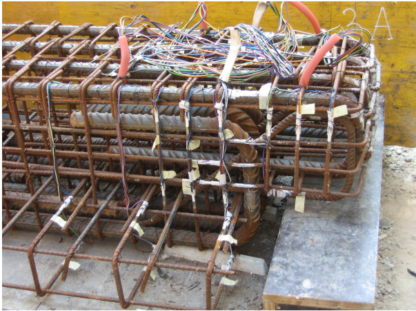
Fig.12. Arrangement of electroresistant tensometers on the reinforcement bars
