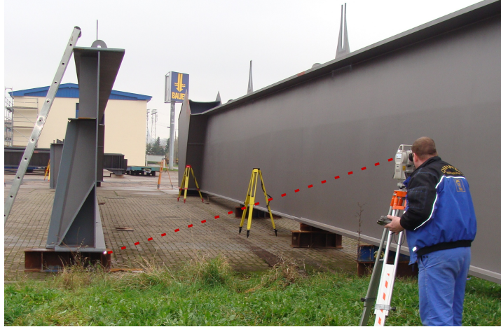
Figure 2: Quality control by measuring discrete points with total station
