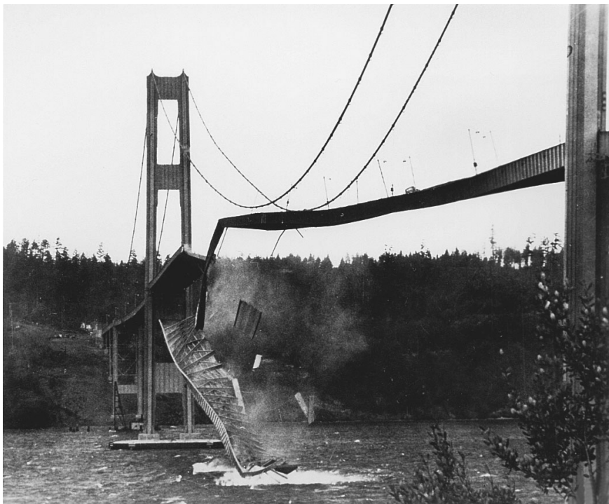
Figure 1.1: The original Tacoma Narrows Bridge collapse, USA [3].
