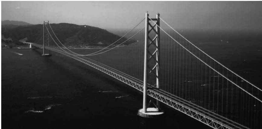
Figure 1.2: Akashi-Kaikyo Bridge, Japan [5].
