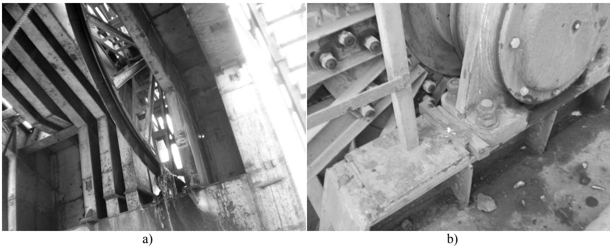
Figure 6: The sub-pulley structures of the upper sub-pulley platform: a) View from below; b) Resting nodes of the guide pulley
