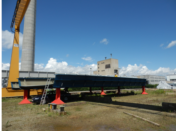
Figure 4.2: The bridge superstructure [26]
