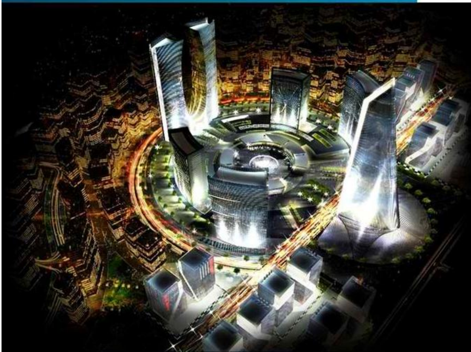
Plate 7.12: The New Eko Atlantic City Project in Lagos under Construction
