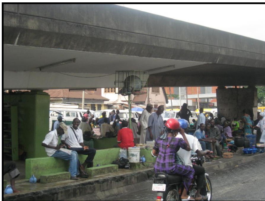
Plate 7.2: Some Lagosians carrying out their daily activities under a highway bridge in Lagos, where some of them sleep
