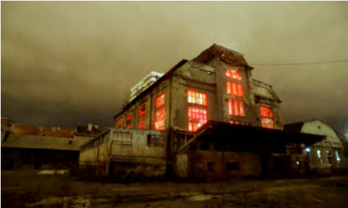
Light installation in the Badel factory building
