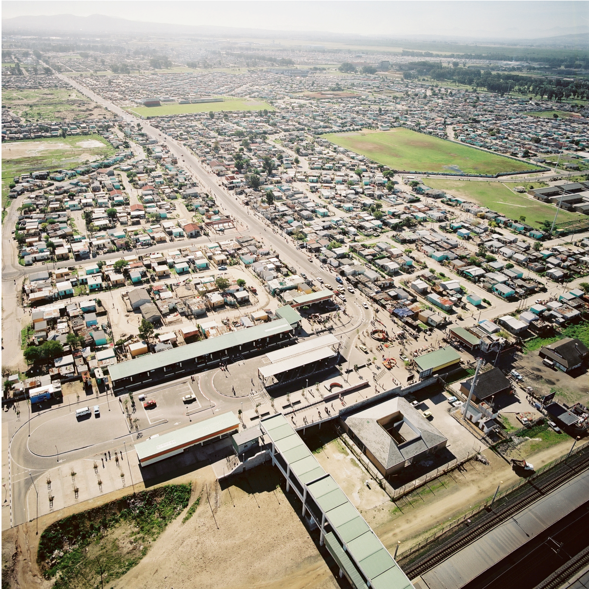
Figure (46) Source: Perrin, 2008. Du Toit & Perrin in Association. Aerial photograph of the Philippi interchange after completion. The Railway bridge (South), Station forecourt with the Taxi rank (middle) surrounded by the trading facilities (North, East).
