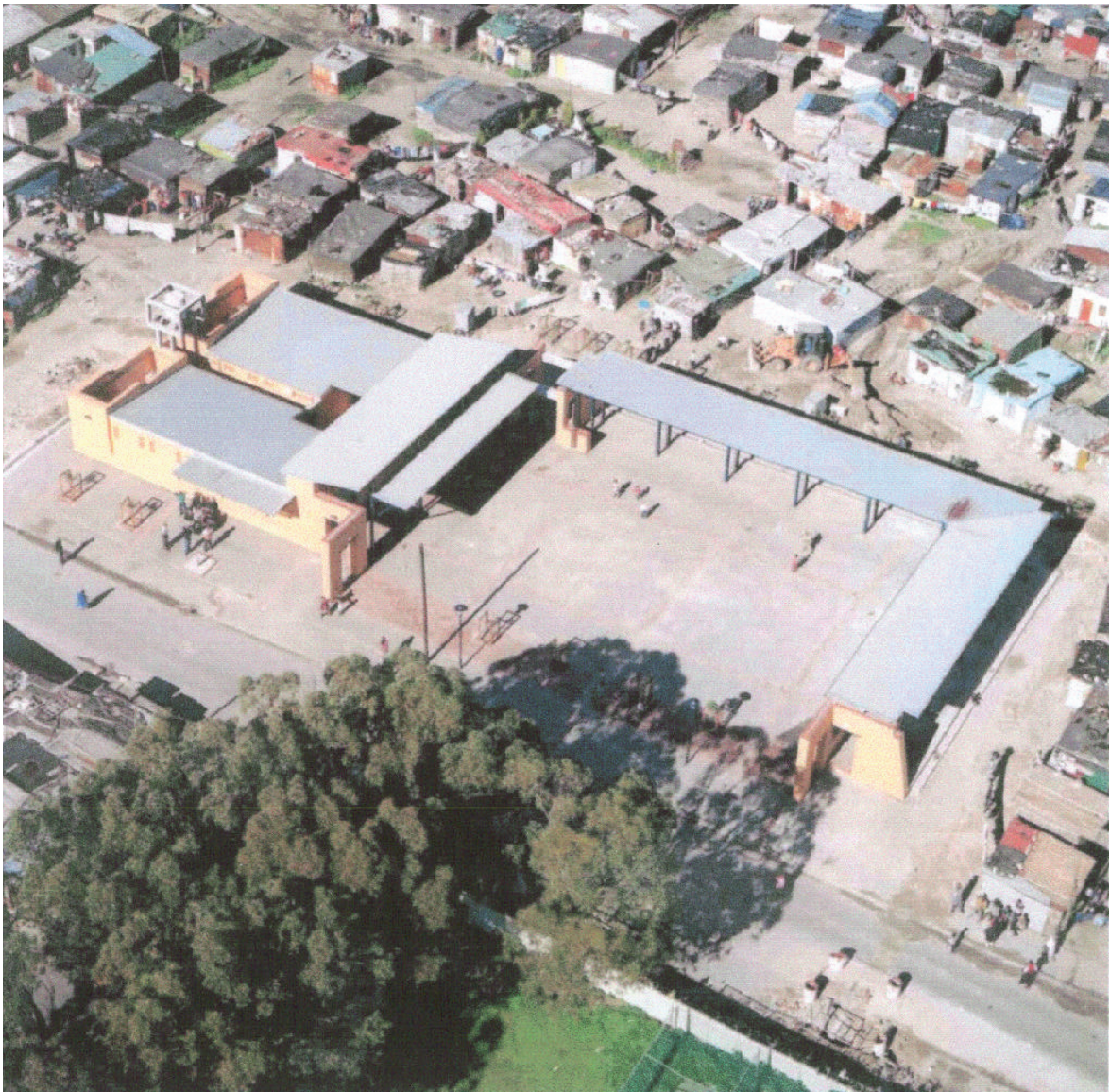
Figure (66) Source: Cape Town's report for the CIA and SAIA Merit Awards (2003). Aerial photograph of the Public Bathhouse surrounded by informal shacks and formal housing before it became vandalised and destroyed.
