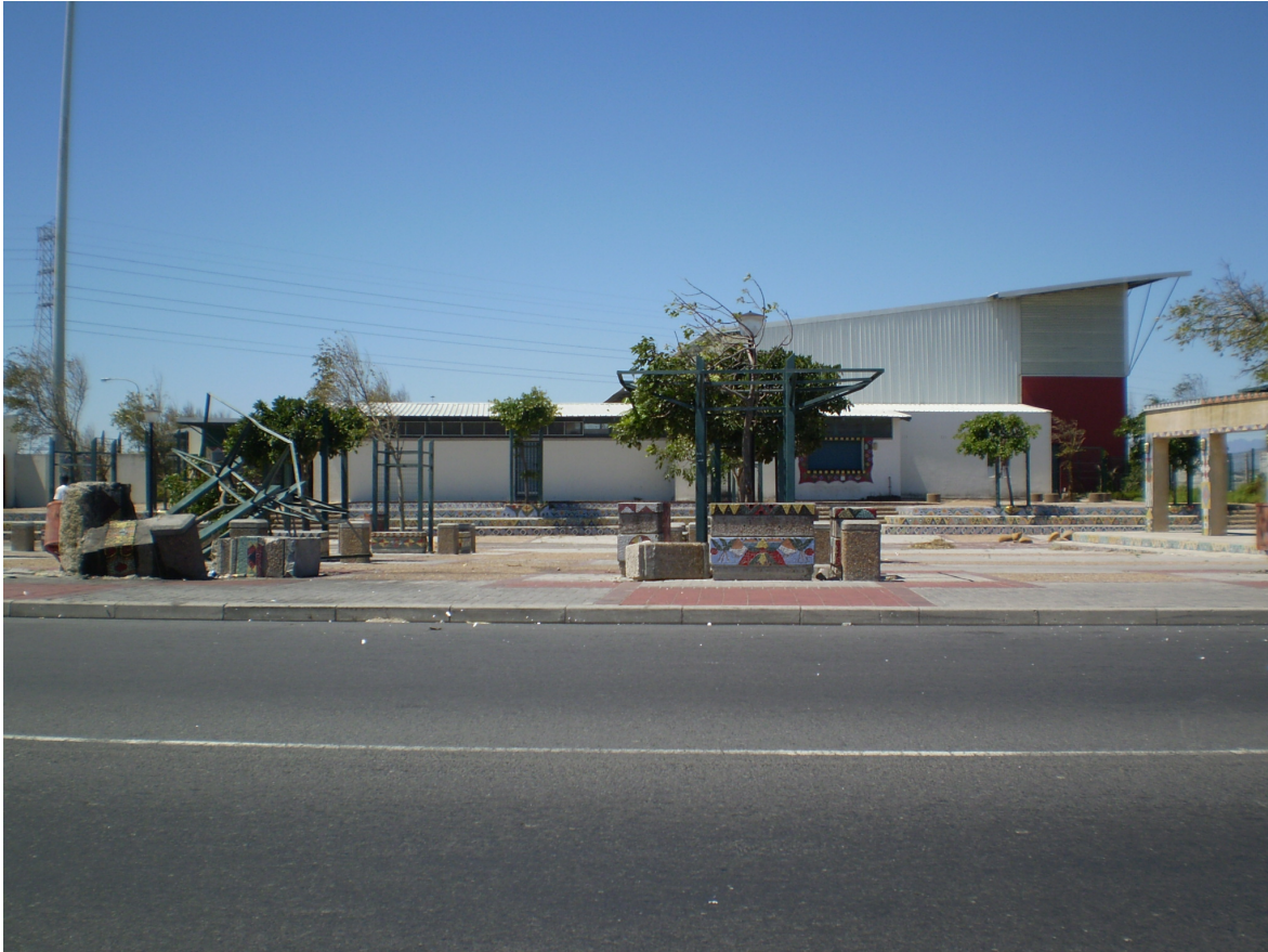
Figure (53) Source: Photograph by author, Philippi Grand Parade project, West elevation, Site visit 19/02/2008.
