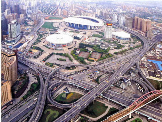
Picture 4-11 Shanghai Elevated Roads 申 (shen) Pattern
