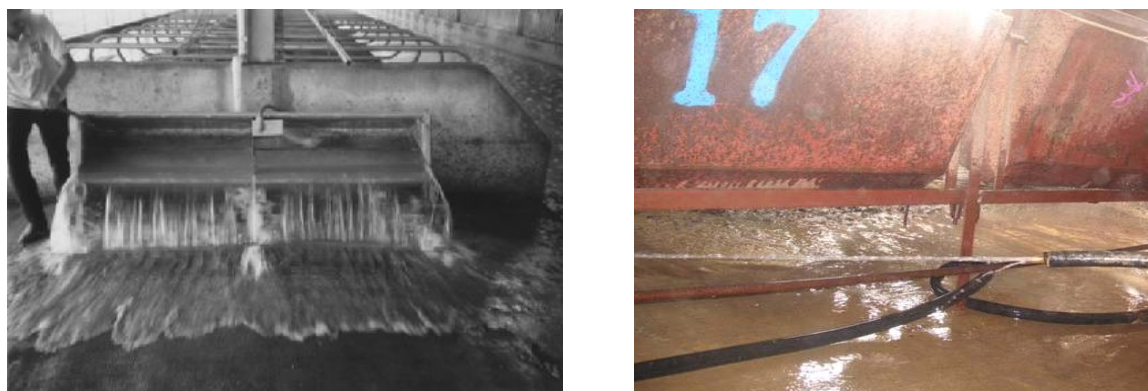
Fig. 4.4: Water valve (left) and pipe (right)
