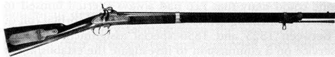
Figure 9 U.S. Percussion Rifle Model 1841 (pattern piece) designed and manufactured at the Harpers Ferry armory. Source: Collections of the Division of Armed Forces History, National Museum of American History. Smithsonian Institution Neg. No. 73-312.
