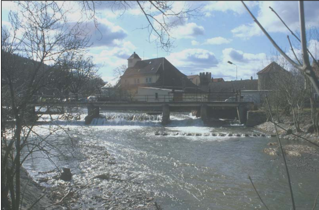
Figure 2.3: A picture of the dam investigated in this study. (View from the site immediately downstream).
