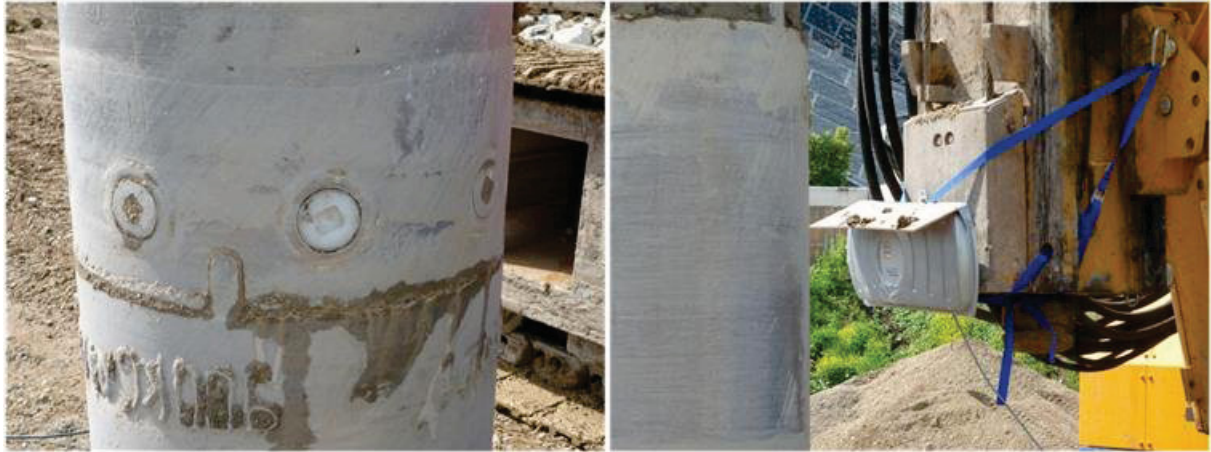
Fig. 5: RFID drill-pipe screw
