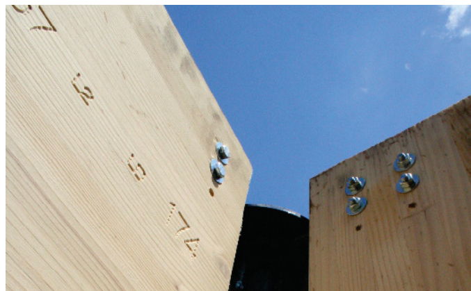
Fig. 9: coded timber panels and different straps
