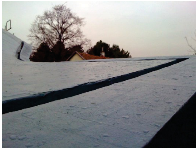
Fig. 5: gutters are completely integrated into the skin
