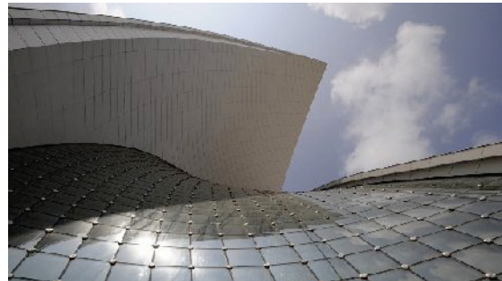
Fig. 10: Close-up of Glass Curtain Wall
