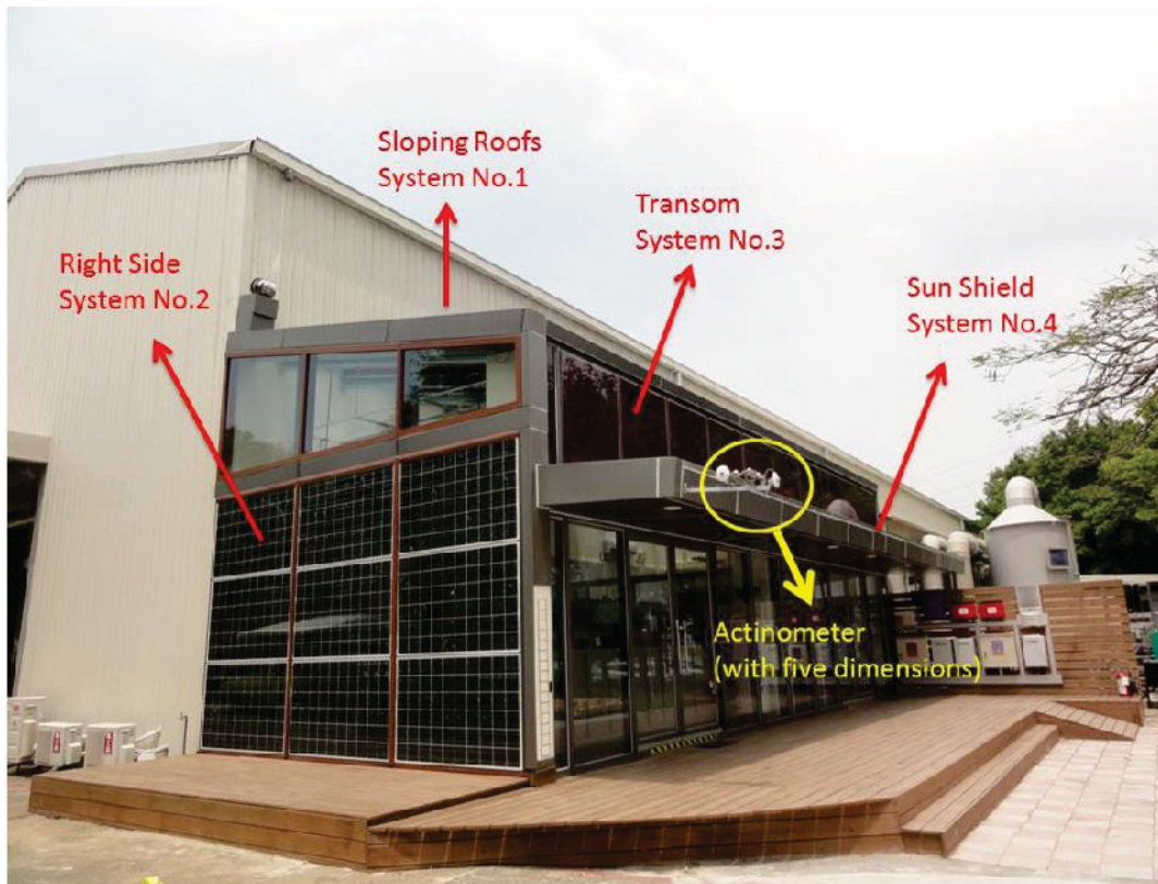
Fig. 2: BIPV Experimental House.
